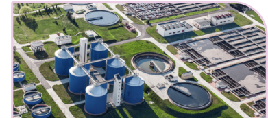
SEWERAGE TREATMENT PLANT
